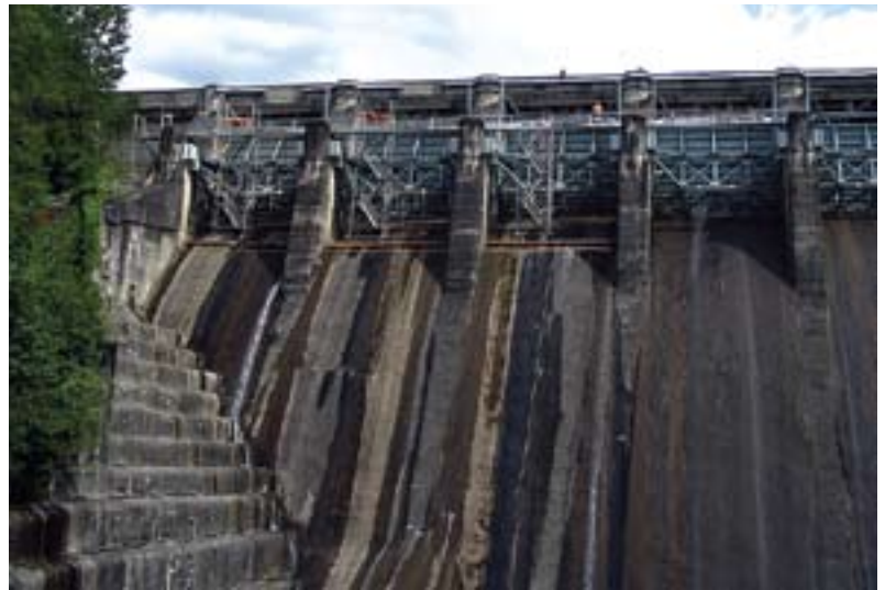
View of Ruskin Dam with temporary access installed at Bays 1, 2 and 3
