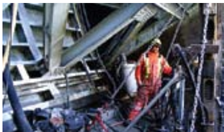
Drilling atop crest block directly beneath gates
