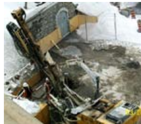
Installing sleeve pipes inside the limited-access site
