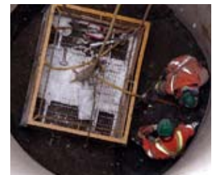
Advancing the steel liner through grout-consolidated soils
