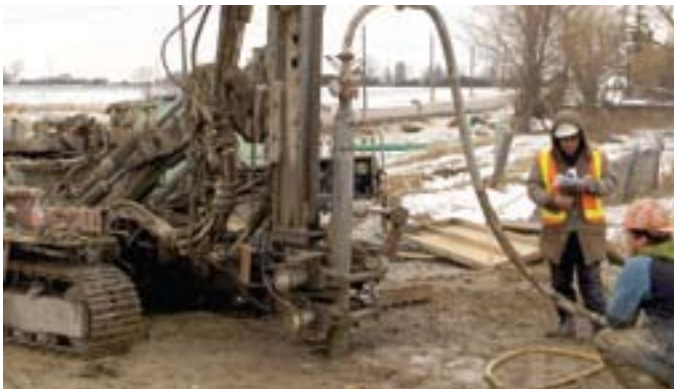
Compaction grouting in progress
