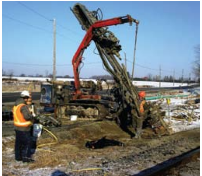
Double-head drilling to install grout casings
