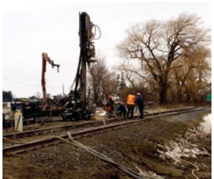
9th Line compaction grouting site
