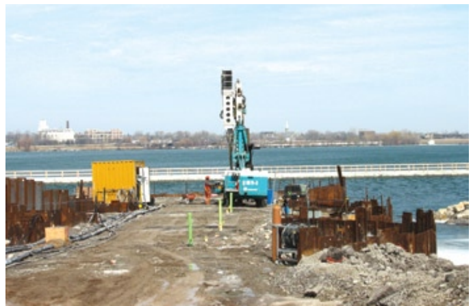
Drilling of 80-metre deep grout curtain holes from atop cofferdam rock fill
