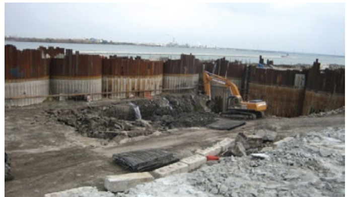
Excavation of intake shaft in progress – November 2007
