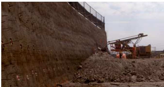
Drilling soil anchors at the eastern arm of the wall
