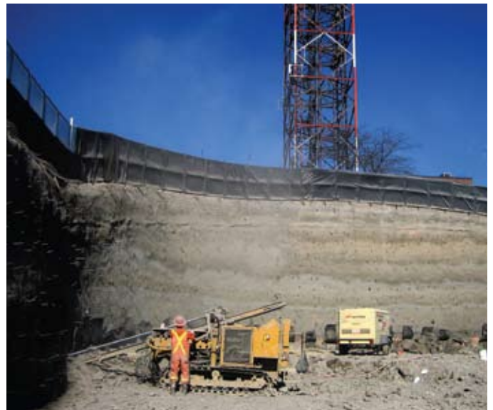
First phase of wall construction nearing completion
