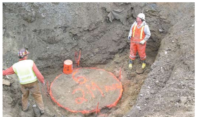
Exhumed jet grouted test column showing 2 metre diameter
