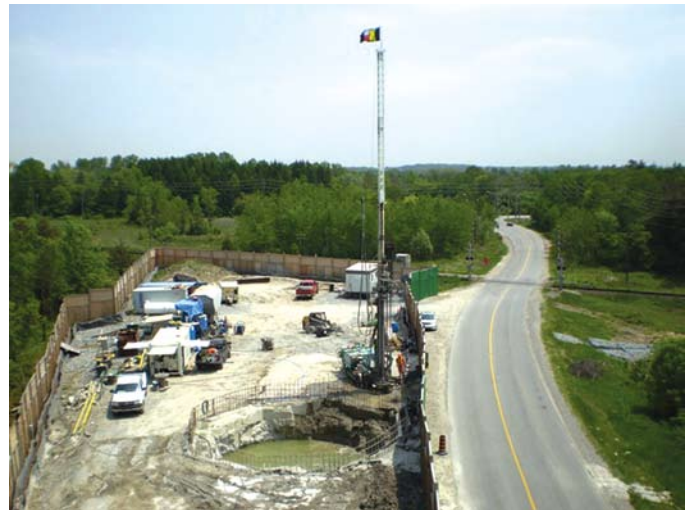
Jet grouting at Shaft #2, looking east along 16th Avenue
