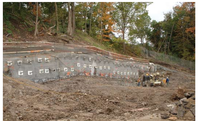
West wall cut beginning to take form
