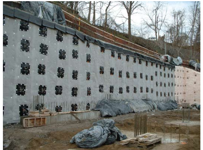
Completed anchored shotcrete wall with waterproofing and studded plates
