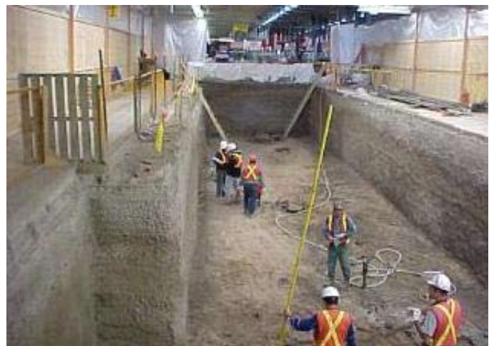
Pit shoring complete, ready for floor slab construction
