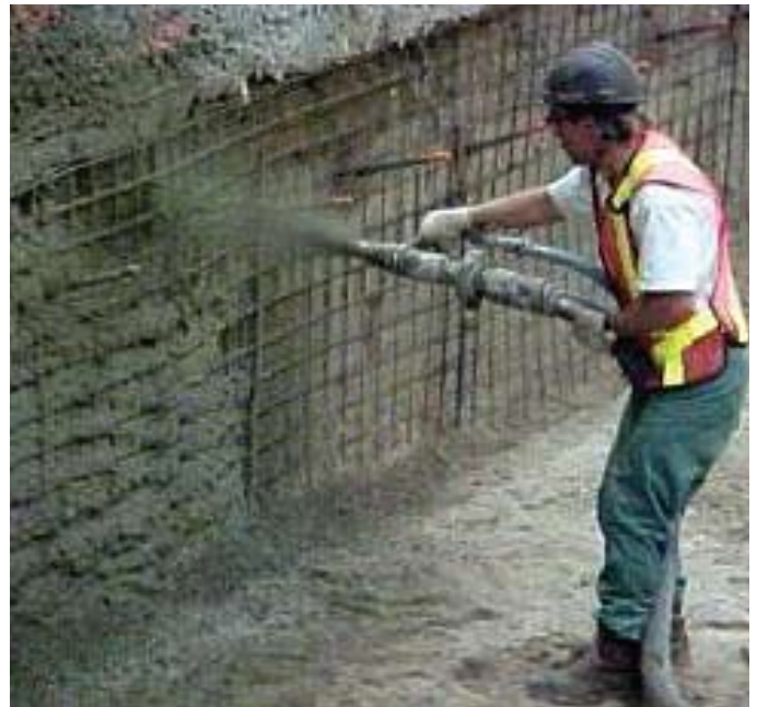
Application of shotcrete to the excavation face at bottom bench
