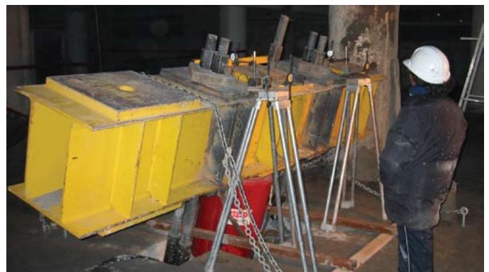
Load testing of a production micropile to 4000 kN applied compression load
