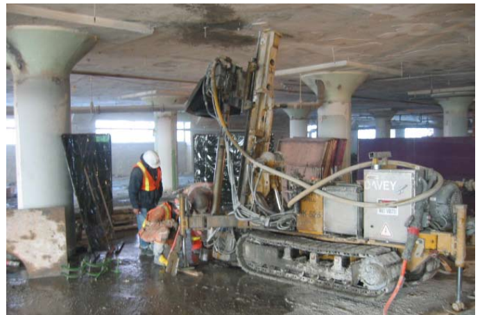
Electric drive drill working in just 3.4m headroom
