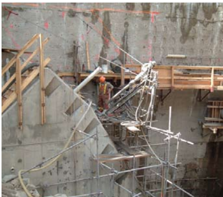
Rock anchor drilling at Plinth B using mast-only drill set up
