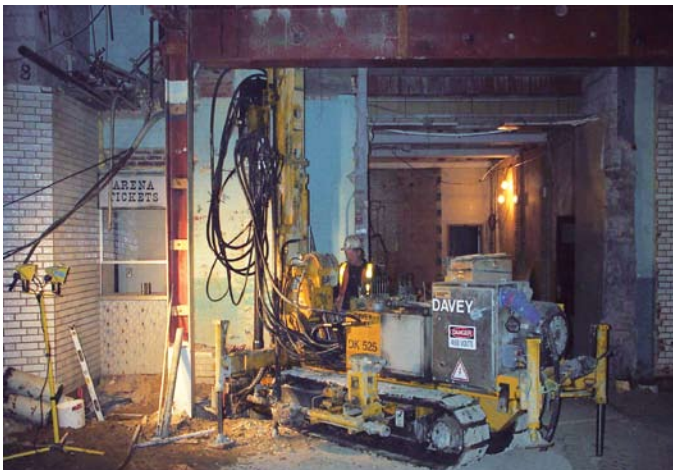
Micropile installation in low headroom beneath south grandstand
