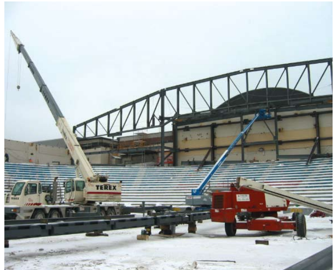
The first of nine major trusses being installed in April, 2003
