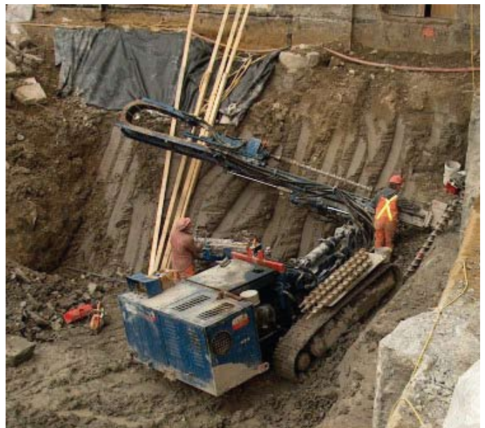
Drilling of soil anchors, east elevation
