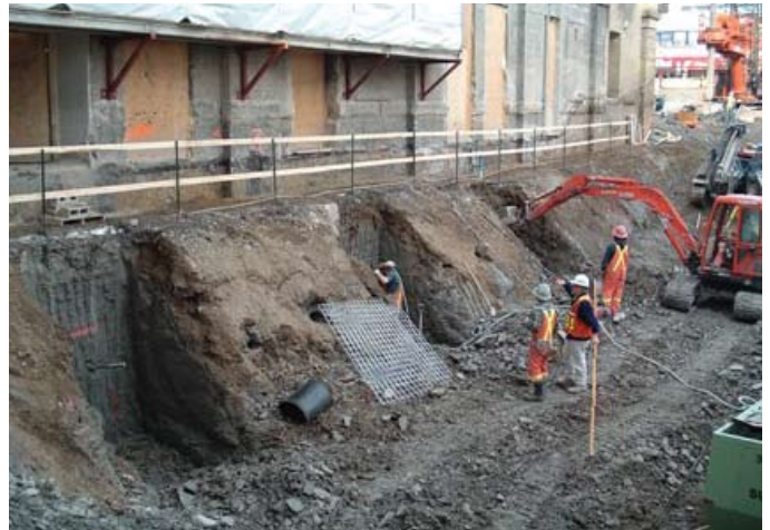
Anchored shotcrete progress, west elevation
