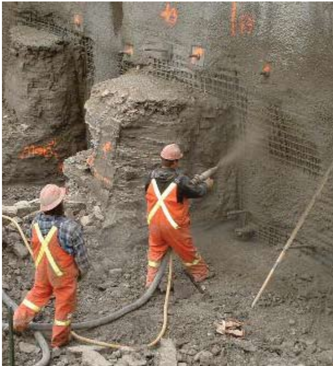
Application of shotcrete at east wall, third bench
