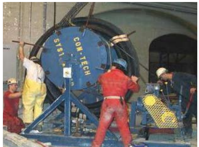
Rock anchor installation using an off-coiler
