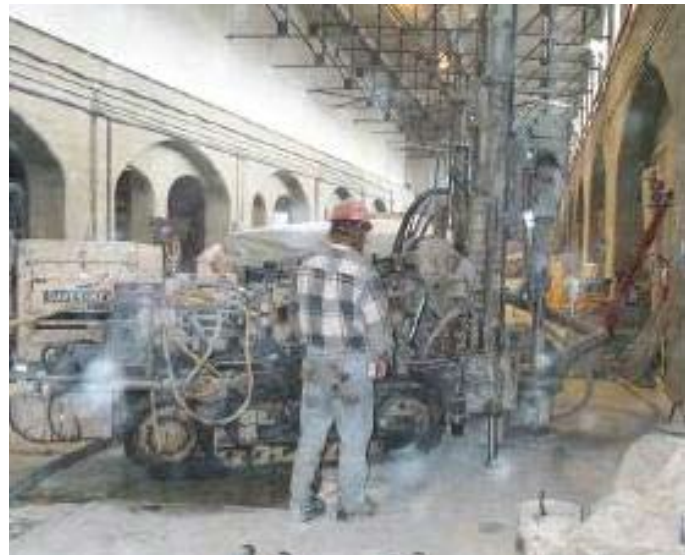
Drilling inside the powerhouse
