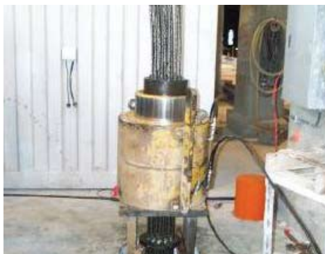
Multi-strand rock anchor in the midst of proof tensioning
