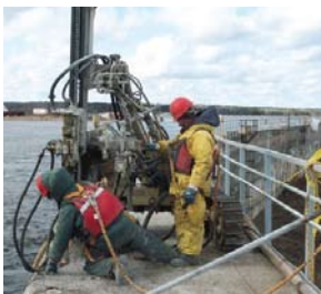
Dowel drilling from atop wall deck
