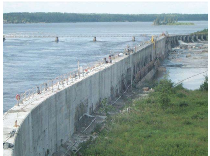
Pointe du Bois – East Forebay Wall
