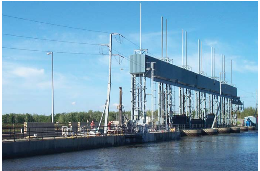
Site view of gravity wall during rock anchor construction
