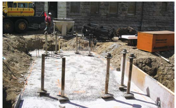
Tension-compression micropile foundations for the West Elevator Core
