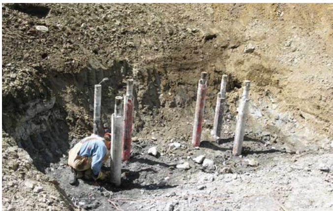
Exhumed micropile tops being prepared for dressing with plates and nuts
