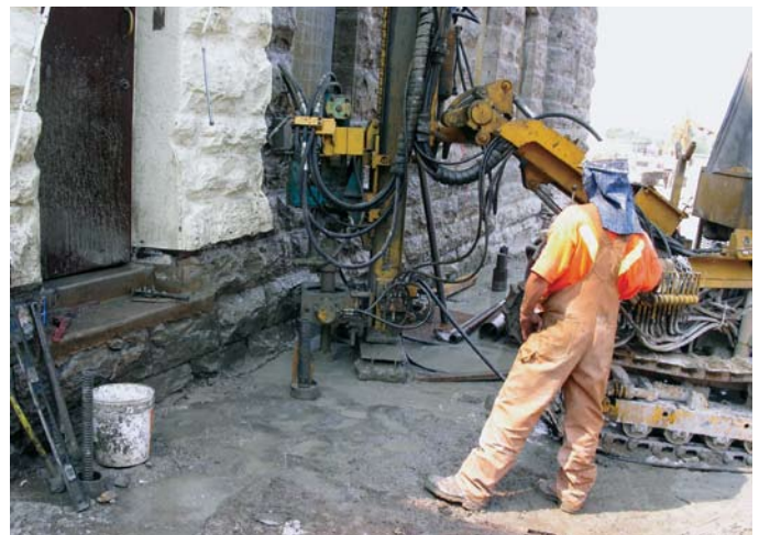
Installation of grout-flushed micropiles within 600mm of heritage masonry walls
