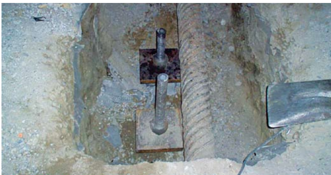
A pile cap excavation showing typical buried conduit conditions encountered
