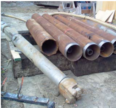
Permanent 273mm diameter steel casings with threaded joints
