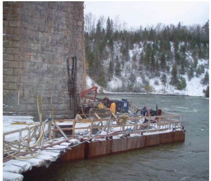
Drilling of micropiles at Pier 2 in November 2004
