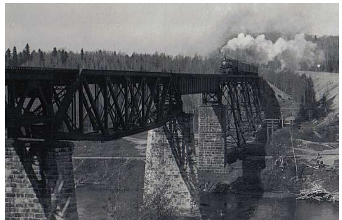
Photo of Nipigon River Bridge taken in 1937 – Piers 1, 2 and 3 from left to right
