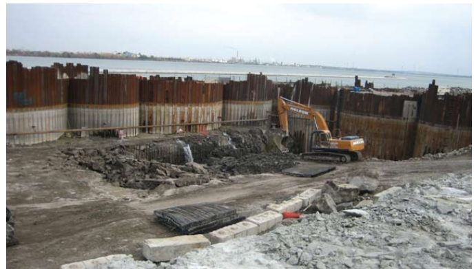
Excavation of intake shaft in progress – November 2007
