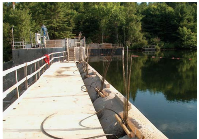
Multi-strand rock anchors as seen after grouting
