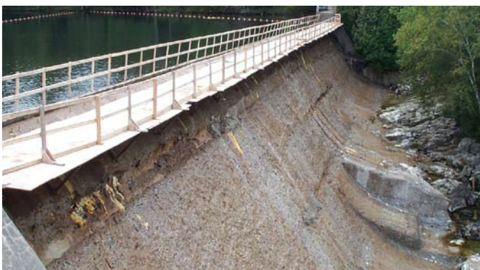
16-metre high dam at Minden GS, as seen at end of 2002
