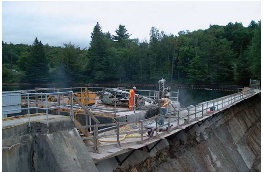
High-capacity rock anchor drilling from barge access
