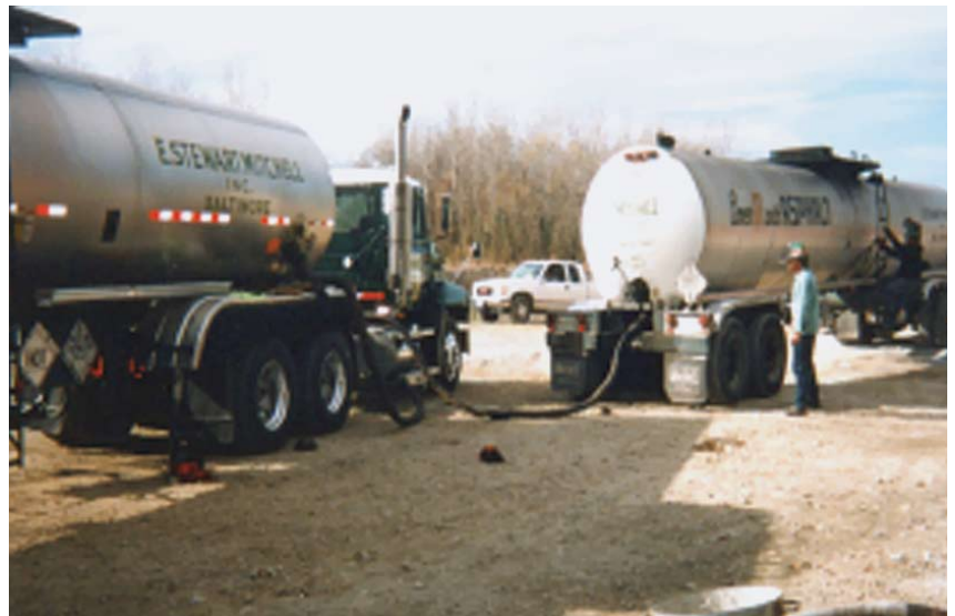
Caravan of hot bitumen tanker trucks delivering grout to site
