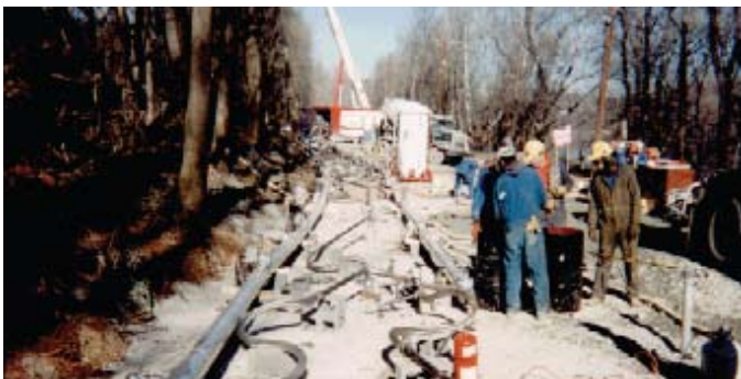
Inflow reduction project site – hot bitumen injection wells in foreground
