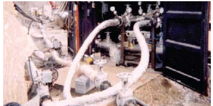
Portable hot bitumen pumping plant in action
