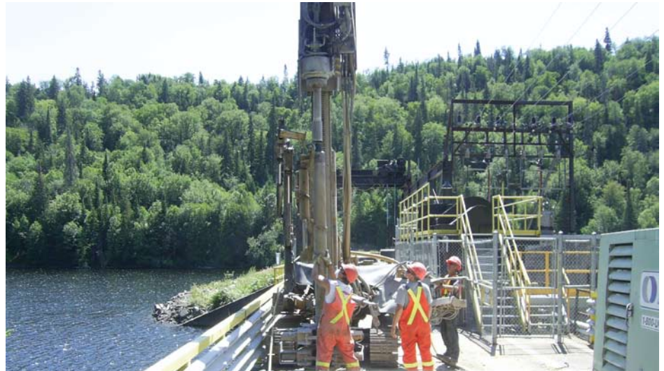
Drilling at Pier 2 at McPhail Dam
