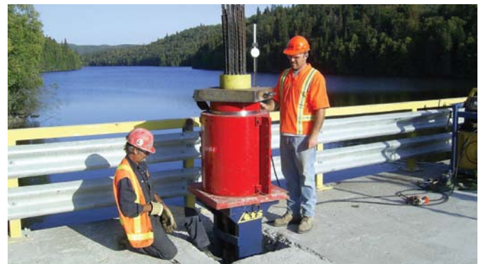
Preparing for performance stressing at Pier 2
