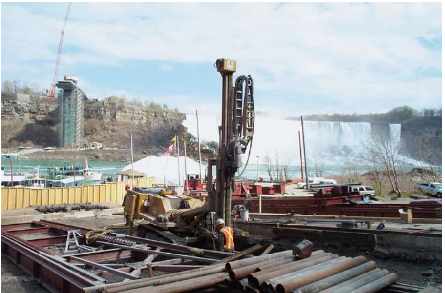
Installation of permanent soil anchors using eccentric overburden drilling technique
