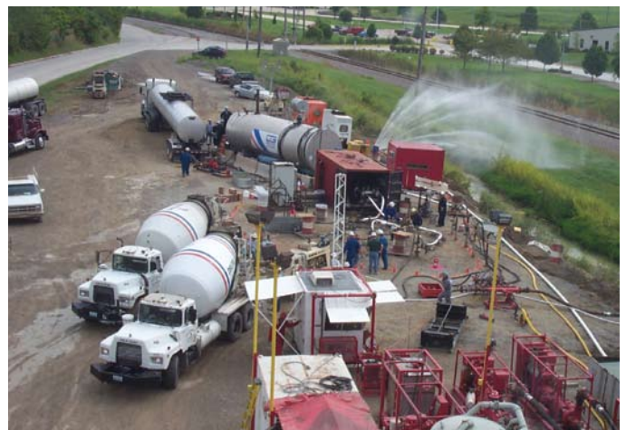
Grouting operation as seen on day of grout injection
