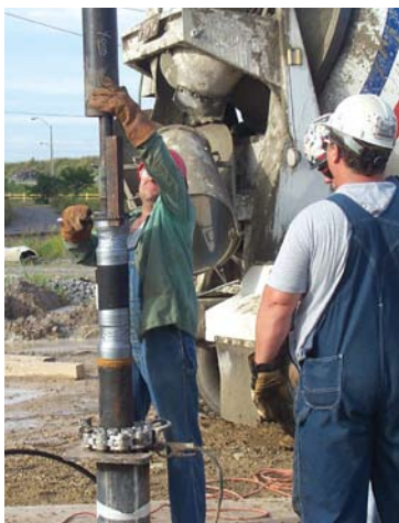
Hot bitumen stinger pipe installation
