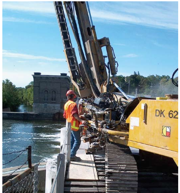
Rock anchor drilling at Pier 12
