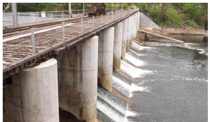
London Street Dam's twelve spillway piers
