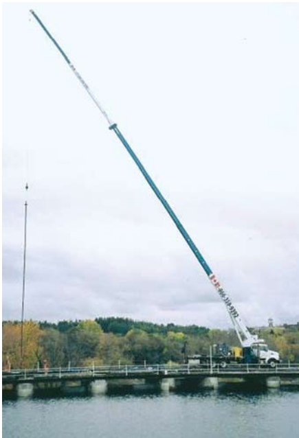
Rock anchor installation by boom truck crane
