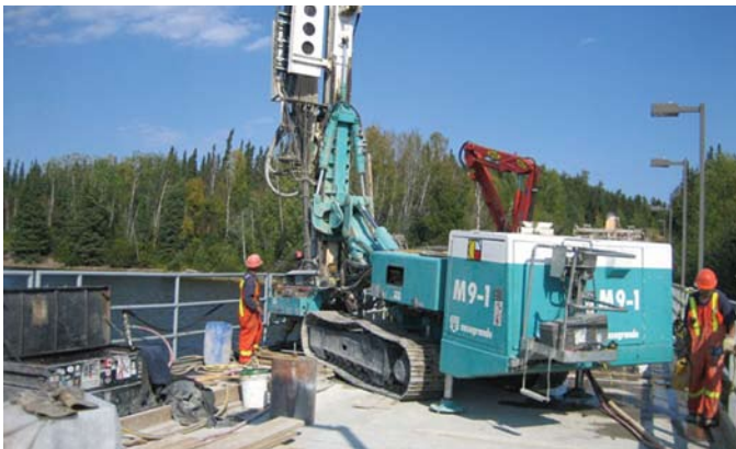
Rock anchor drilling from on top of dam deck
