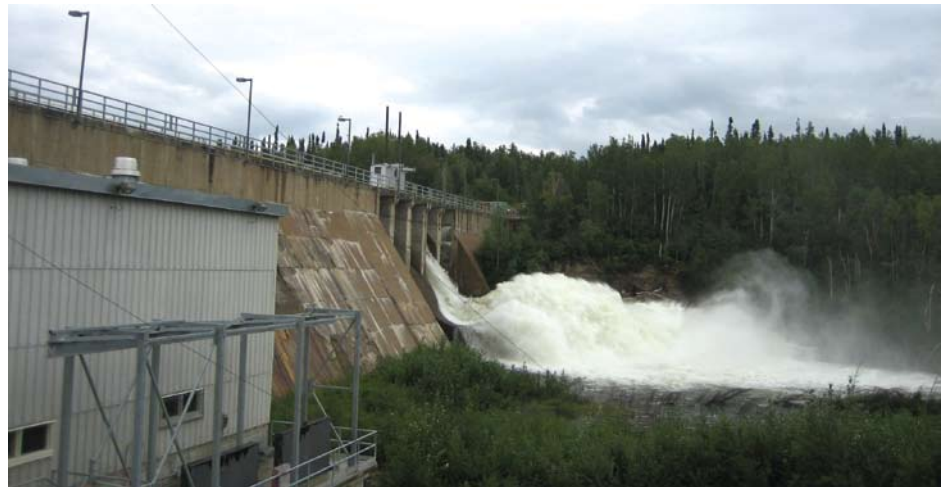
Manitoba Hydro Laurie River Generating Station #2
