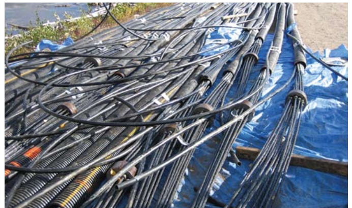
Strand anchors laid out awaiting pick up and installation by helicopter
