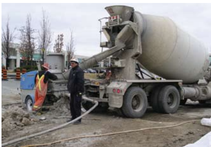
Pumping of low mobility cement-based grout delivered by ready-mix truck
