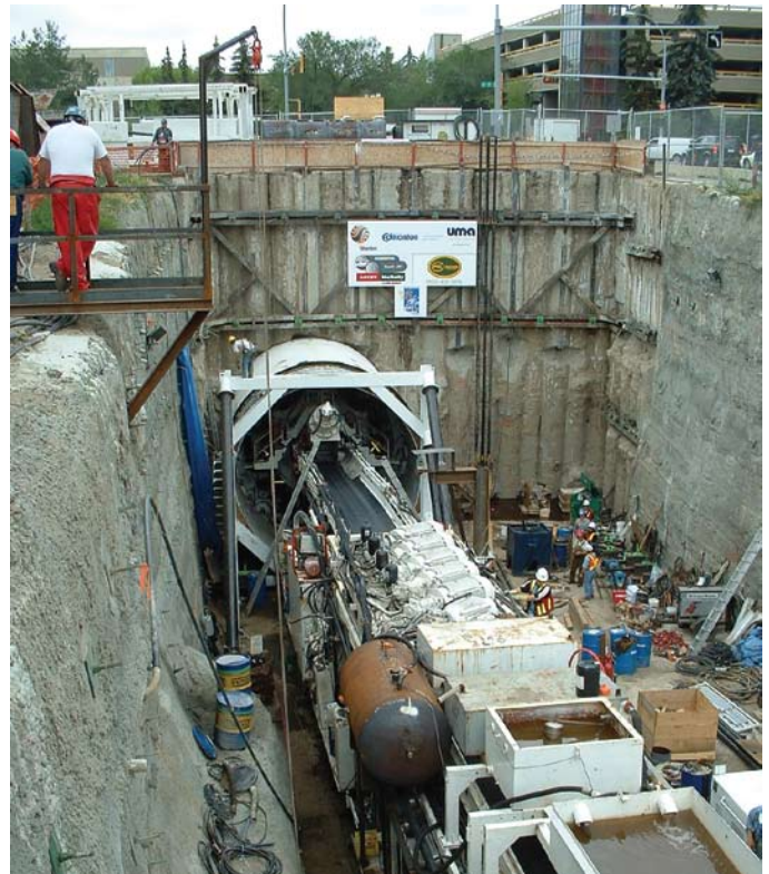
Tunnel boring machine launch shaft south of 87th Avenue
