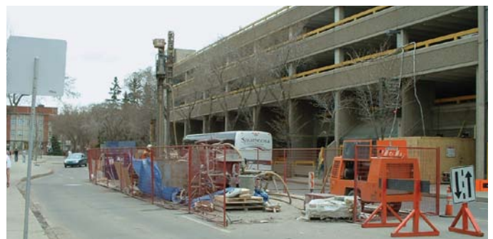
Installation of grout delivery pipes from 114th Street
