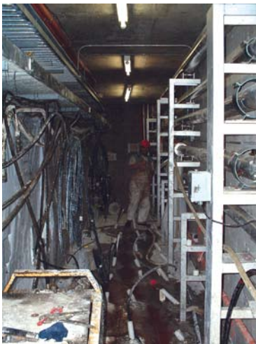
Grouting in progress from inside the utility tunnel
