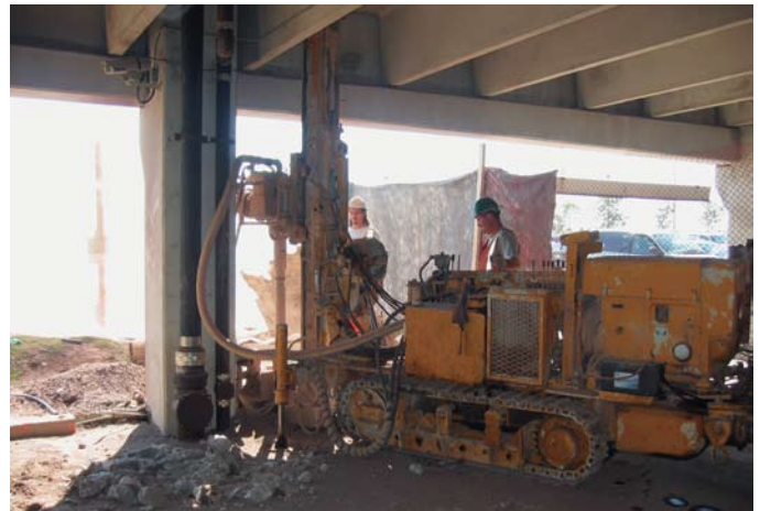
Low headroom micropile construction at Column A-4
