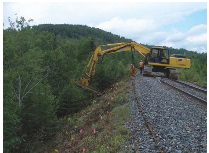
Soil nailing at Latuque, Quebec
