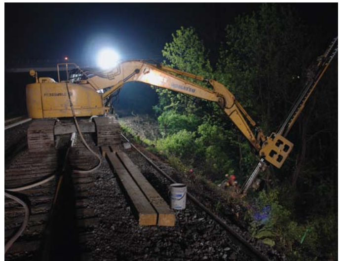
Sunfish Pond: zero-clearance rig installing soil nails during night shift
