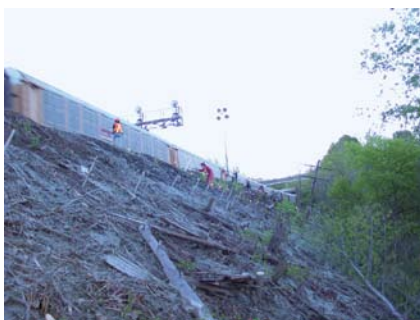
Sunfish Pond: south slope of rail embankment with new soil nails
