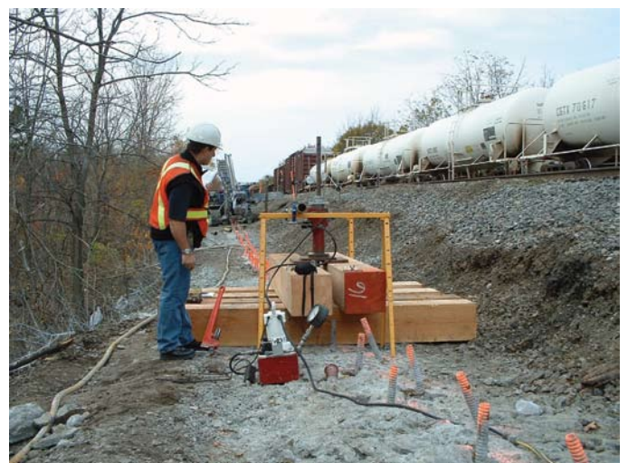
Micropile load testing
