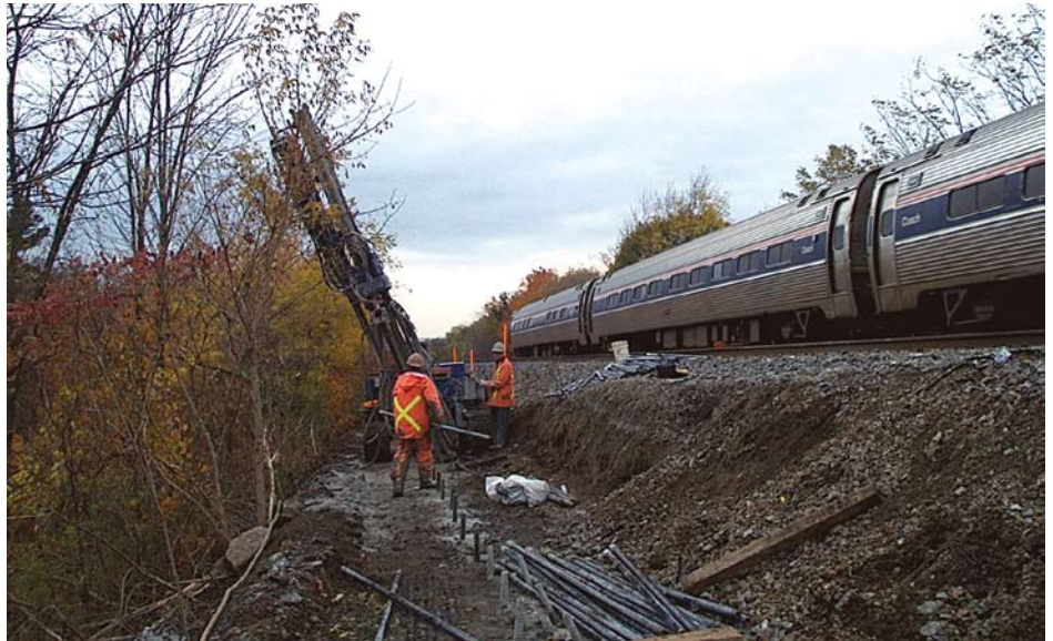
Micropile installation with fully maintained rail service
