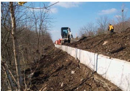
Final re-grading after cap beam construction
