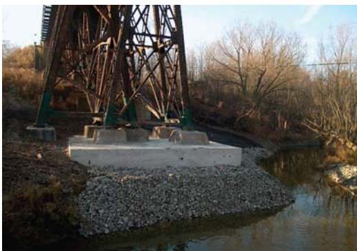
New ring beam encapsulating rehabilitated pier grouping
