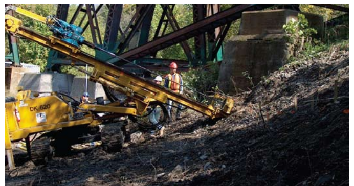
Soil nail installation at south creek bank
