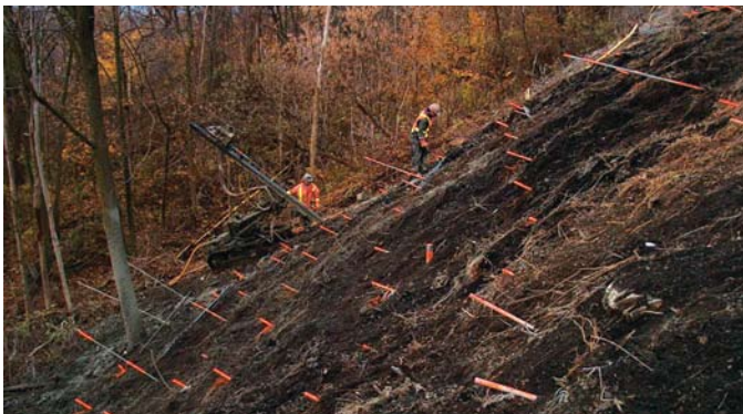
Soil nail construction ongoing with completed soil nail array in foreground
