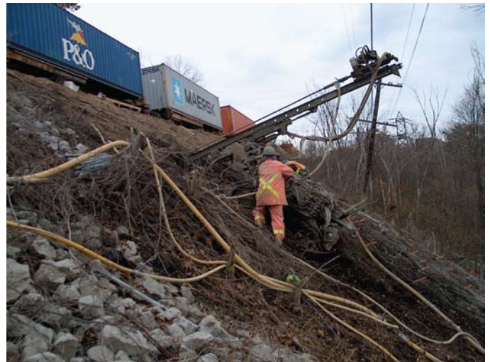
Soil nail construction proceeding while full service of railway is maintained
