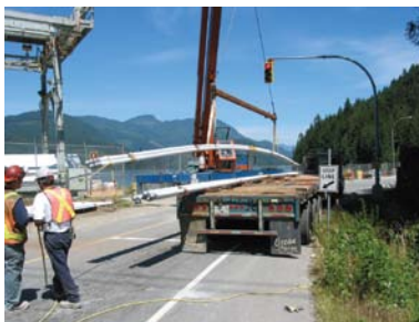
Delivery of 19-metre long triple-bar rock anchor segments
