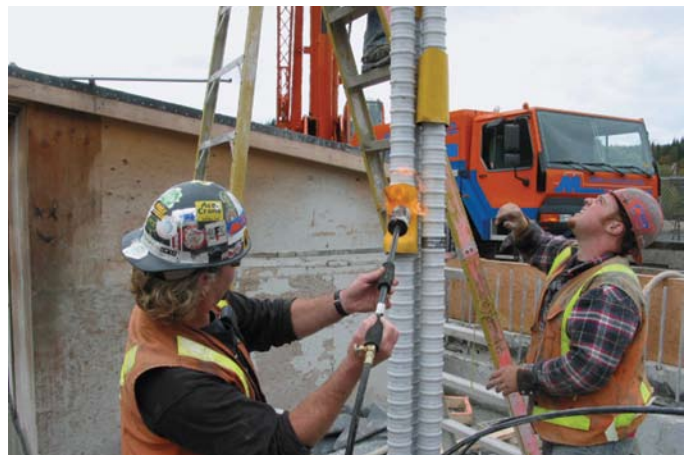
Heat-shrink sleeve being installed over a single-bar field splice
