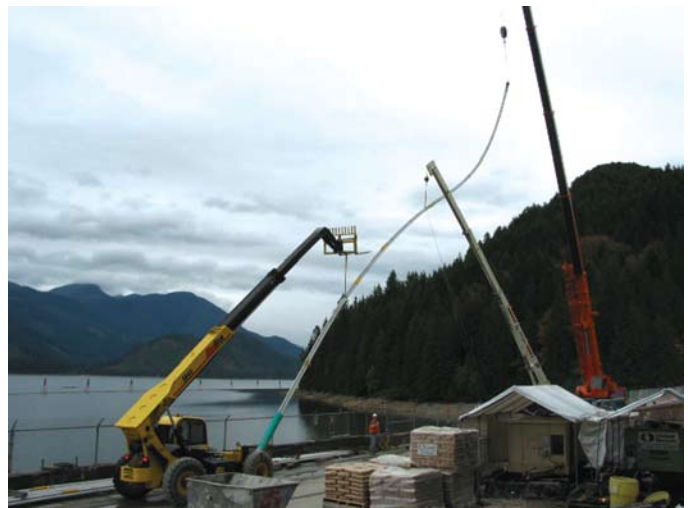
Hoisting of triple-bar rock anchor segment using 3 independent hoists
