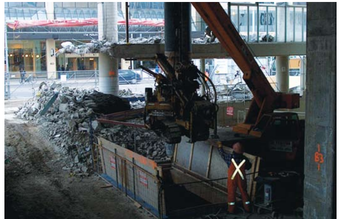
Hoisting the drill into the sub-basement in the midst of tower demolition above
