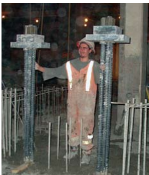
Triple-bar reinforced tension micropiles for the new elevator core foundation
