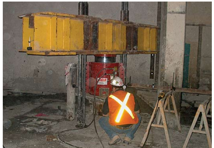
Static compressive load testing in the sub-basement
