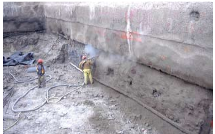
Applying shotcrete at C-level bench
